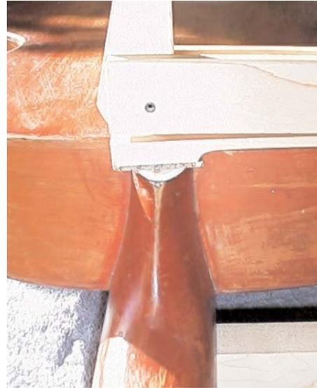
The original plastic neck heel cap had been broken many year ago. To replace it, I first slipped a knife under the plastic and popped the cap off, then cut out a small piece of antique ivory, which was nearly the same color as the old plastic, and glued it in place.
